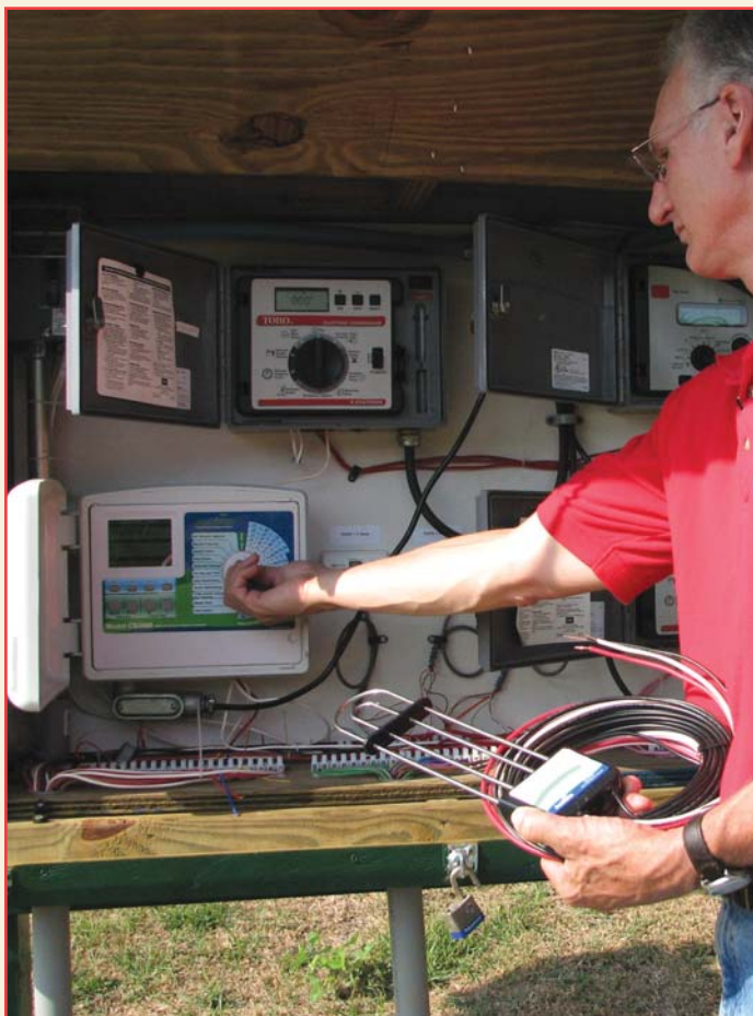
Two of the systems being evaluated have moisture sensors like the one in this photo (here, Dr. Grabow is “adjusting” the “on-demand” system).
